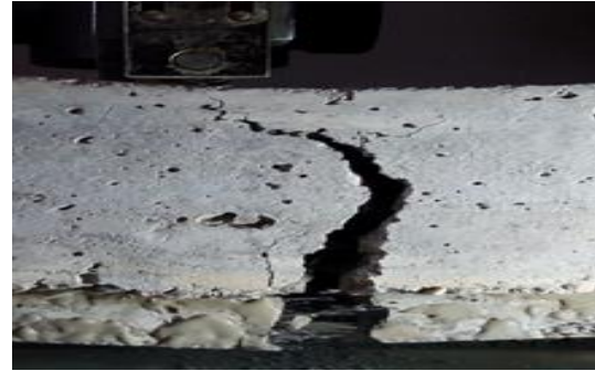
Fig. 10. Expanding the crack and increasing the crack width and bridging action of the fibers in specimen RSWH3PE
