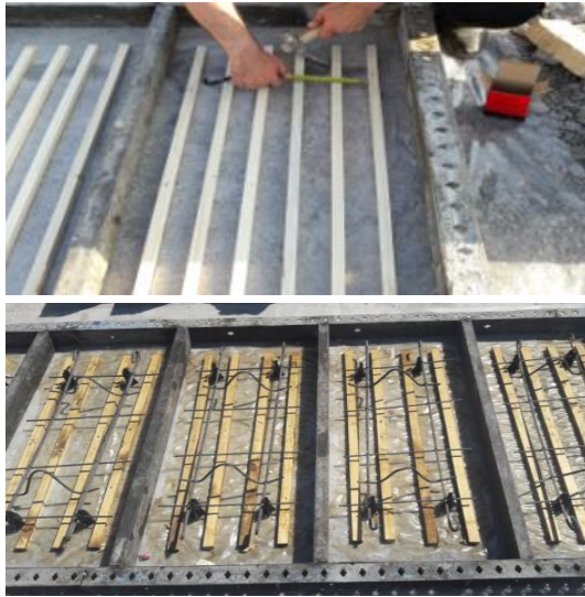
Fig. 6. Arrangement of reinforcement slabs
